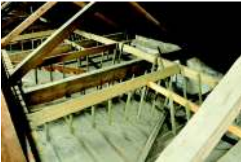
Above the Nave Ceiling
